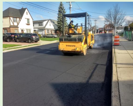
ROAD CONSTRUCTION SUPERVISION
