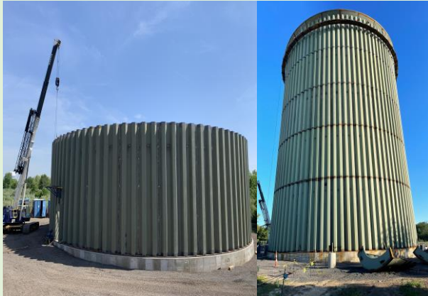
WATER TANK CONSTRUCTION
