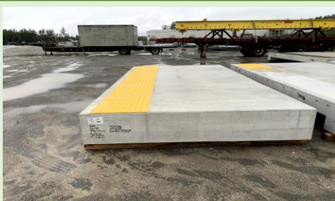
PRE-CAST PLANT INSPECTION
