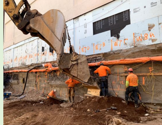
UNDERPINNING INSPECTION
