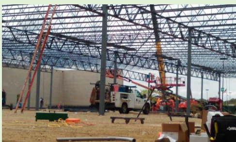
STEEL CONSTRUCTION INSPECTION
